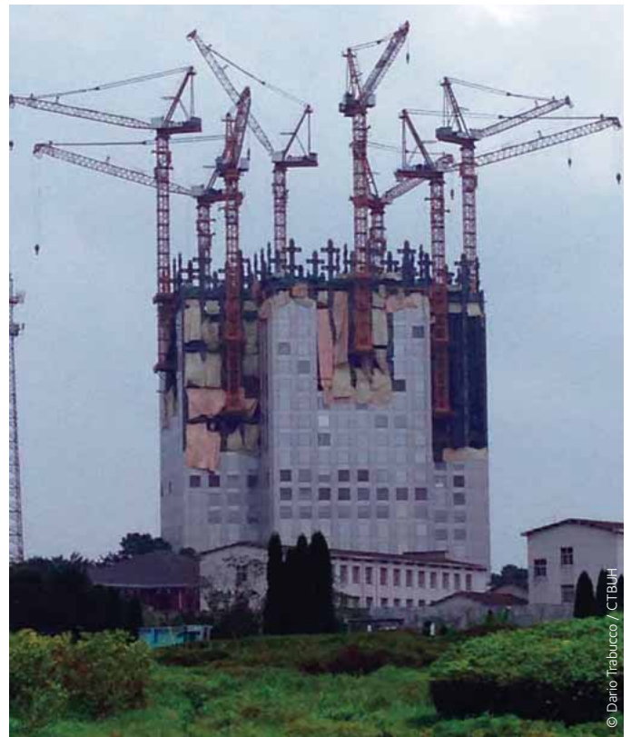
Figure 1.2: Broad J57 Tower, 19 days for 57 storeys, Changsha, China
