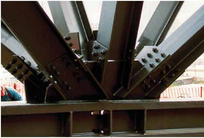
Figure 6.7: Mariner Stadium close up on gusset plates connection in S355 (Gr. 50) with S460 (Gr. 65) beams
