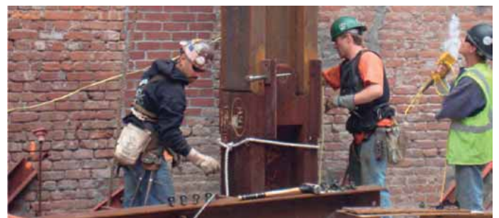
Figure 6.2: Column joint before welding
