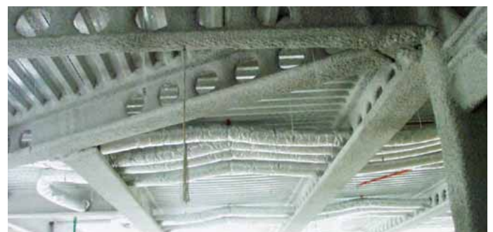
Figure 8.2: Protection by spraying on ACB® beam
