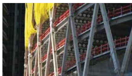
Spray fire-protected diagrid
