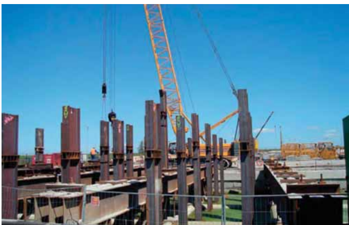
Figure 7.2: Use of HE 800 B with lengths ranging from 33,80 to 38,80m for foundations (Wilhemshaven power plant).
