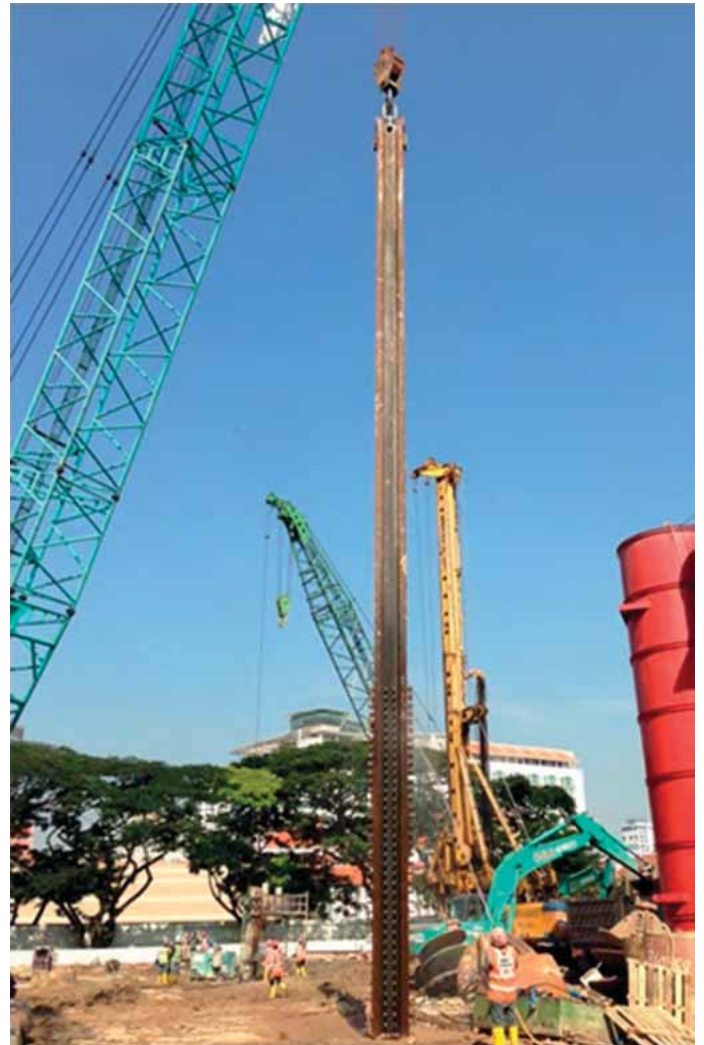
Figure 7.3: 26-metre long foundations for the top down construction method with no splicing required.
