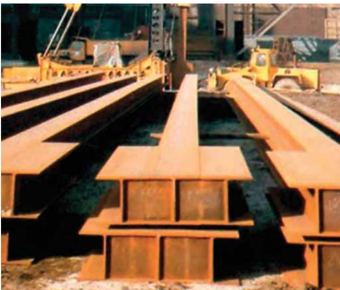
Figure 7.1: Driven piles with reinforcement at the base to increase the cone friction resistance and thus provide support for high loads.
