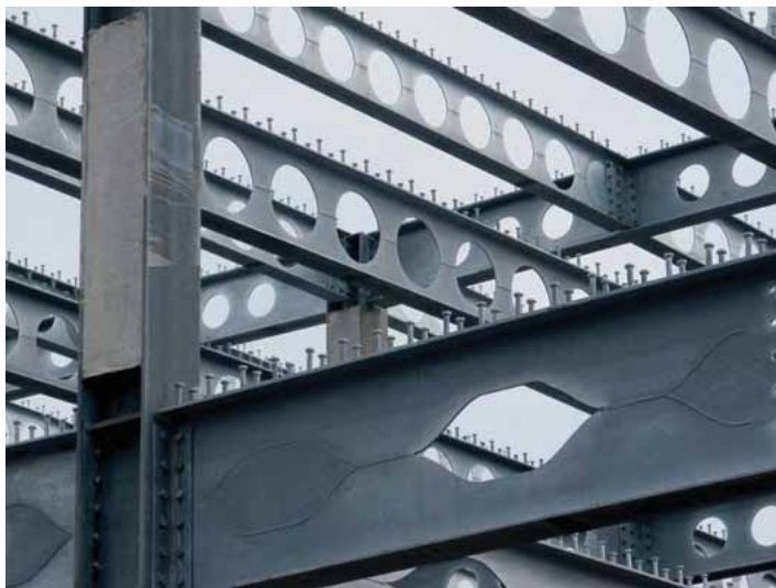
Angelina™ beam with filled openings at support
