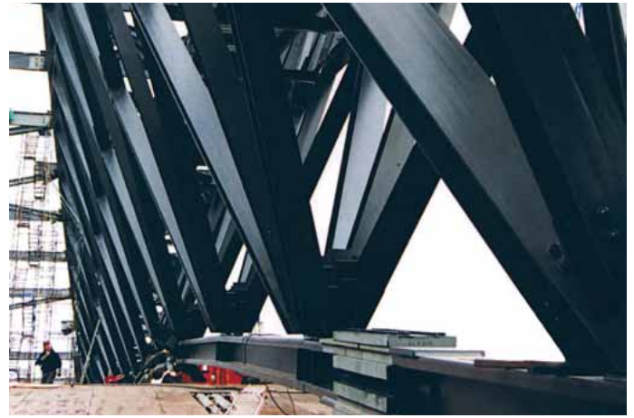
Figure 6.5: Gusset plates connection in S355 (Gr. 50) with S460 (Gr. 65) beams at Mariner Stadium (Seattle)
