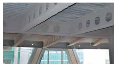
Spray fire-protected beams
