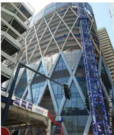
Figure 1.1: Tour D2, half of the weight is carried by exterior steel diagrid, Courbevoie, France
