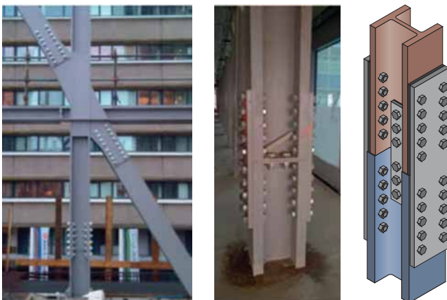
Figure 6.1: Bolted connection of two HD/UC/W columns
